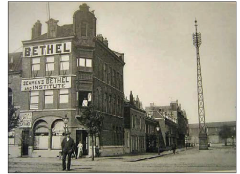
Fig. 10 - Distribution pole in Rotterdam, NL Source: Arnold Abels, Van Houwelingenmuseum Rotterdam, NL.
