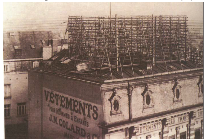
Fig. 3- A derrick on the roof of the Antwerp telephone exchange building
