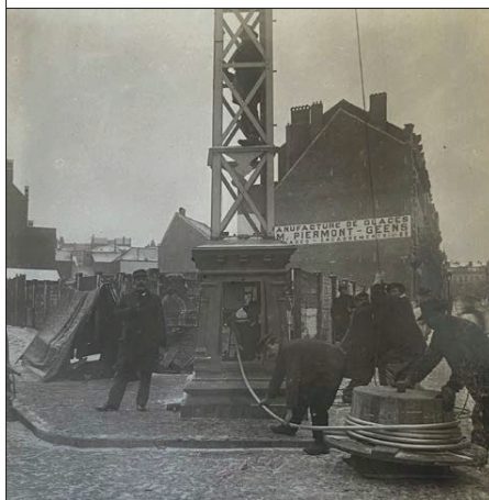
Insertion of a cable into the distribution pole
