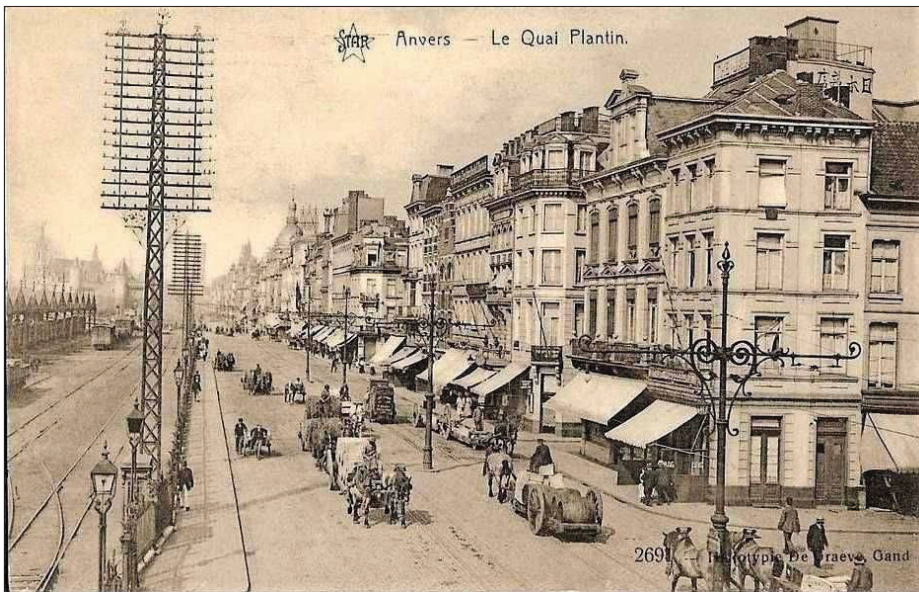
Fig. 1 - Example of aerial telephony wiring in the mid-1890s
