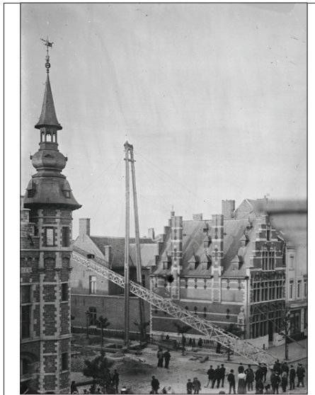
Erecting a distribution pole
