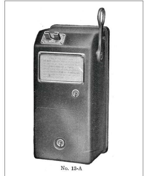
Fig. 6 - Western Electric's coin box 13-A (1908) Contrary to the Gray solution, the Western Electric coin box only had one slot where three different coins could be inserted (nickel, dime or quarter). For each coin a gong was activated either one, two or three times.
