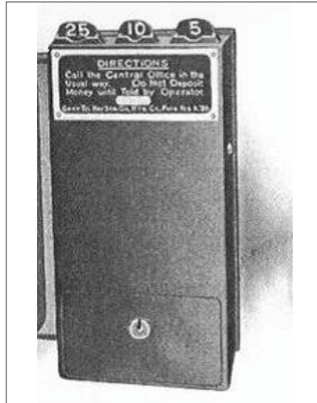
Fig. 5 - Gray's coin box (1912) Gray was the market leader in the USA at the beginning of the 20th century. In their catalogue of 1912, in addition to pay phones, they also displayed coin boxes. At the operator's request it was possible to insert coins. Each slot had its own sound, so that the operator could hear which coins were inserted. Gray was active in the US, but had also distributors worldwide. i.e. BTMC was their distributor in Belgium.
