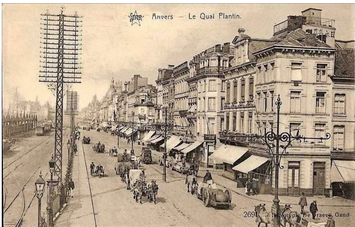
Figure 1: Example of aerial telephony wiring in the mid-1890s
