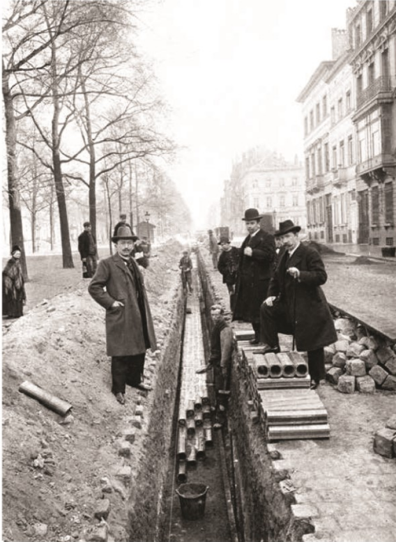
Figure 6: Installation of underground cable in Brussels (+/-1900)
