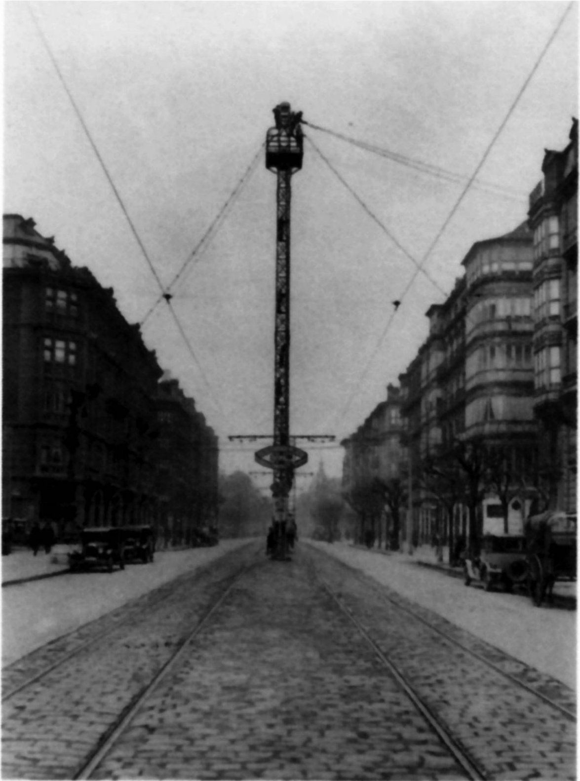
Figure 4: Iron distribution pole in Bilbao, Spain (1928)
