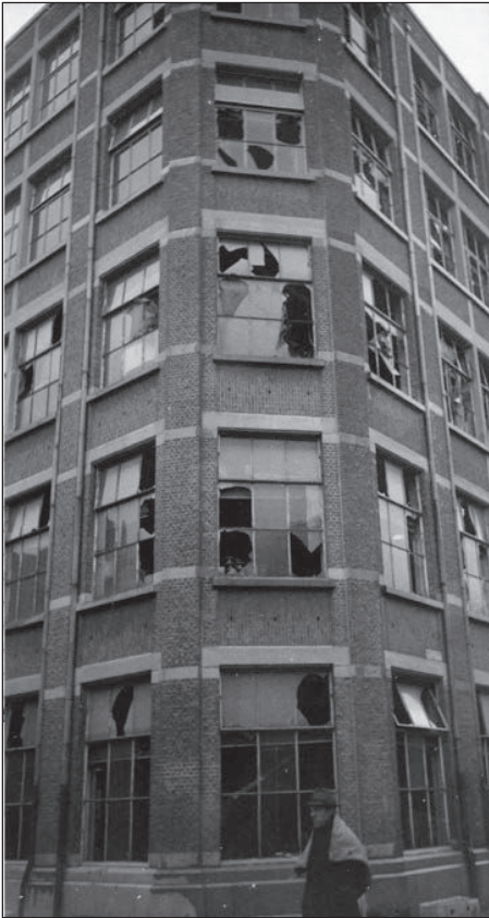
Figure 11: "Collateral damage" in November 1944 due to a V2 bomb. Source: ATEA archives.
